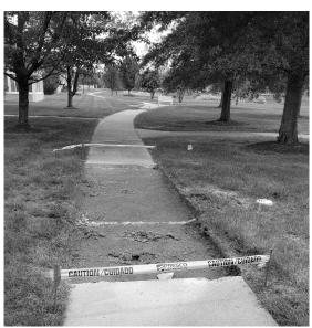
First the existing sidewalks were removed. Gravel fill was added to the saturated soil to facilitate water flow. Drains and piping were added next in order to carry water to the new drain field headed to the pond.
