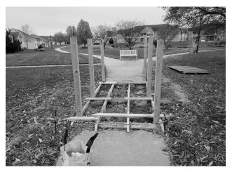
Wheeled vehicles were expected to use the bridge, so guard rails were necessary to keep vehicles from rolling off the sides and to prevent bungy jumping off the bridge.
